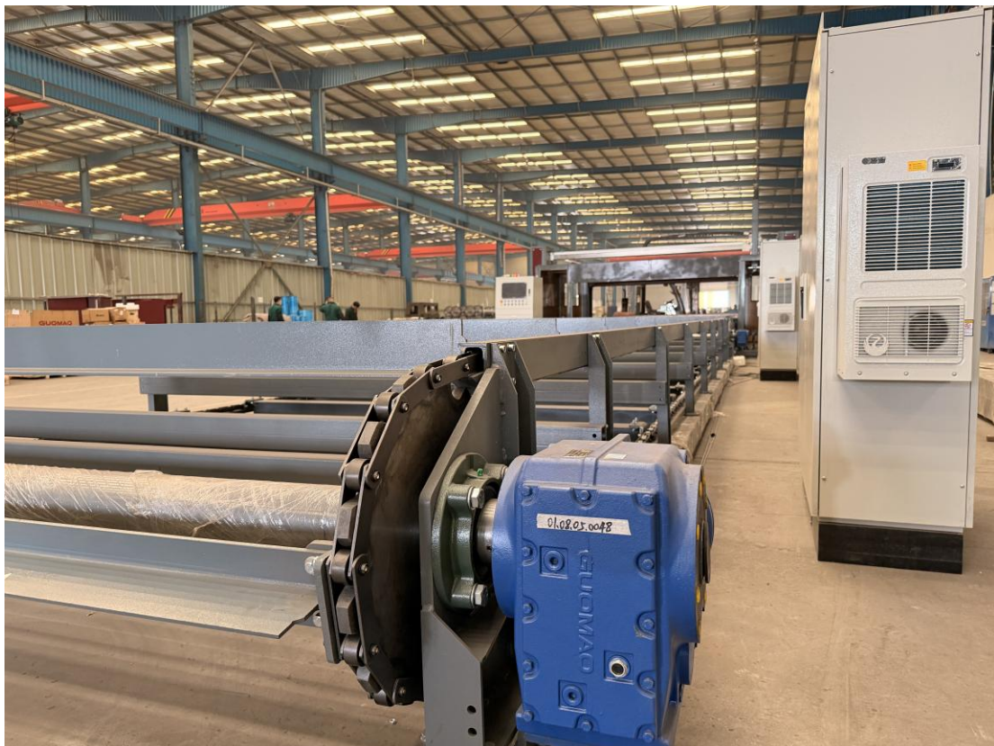
Drying area conveyor syste
